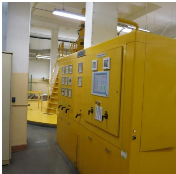
Figure 30. American Governor Digital Governors Installed Circa 2012
