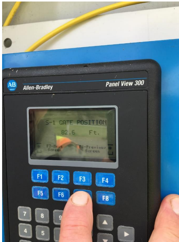
Figure A2-4. Panel Outside of PH Showing Gate Position in EFL Entrances.
