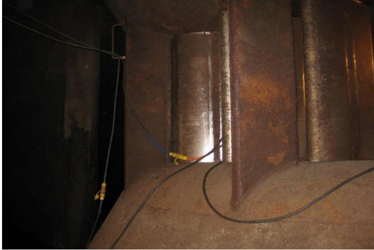
Figure 22. Wicket Gates and Stay Vane in Good Condition
