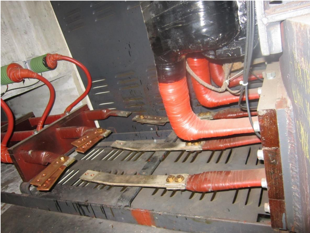
Figure 11. Main and Neutral Leads
